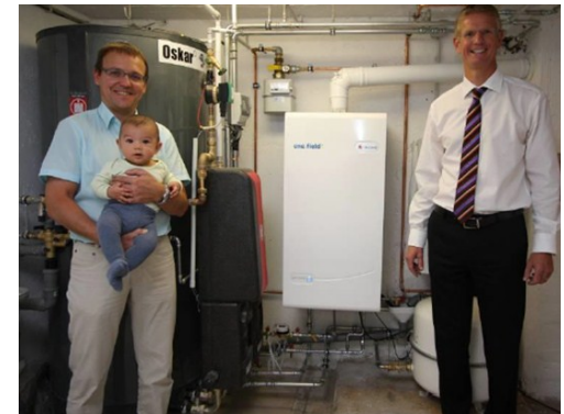
Installation of the Elcore 2400 system at family Aberl (Munich region)
